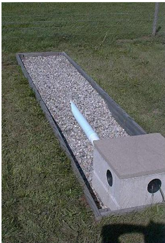
Rock and pipe filled trench at a demonstration site
