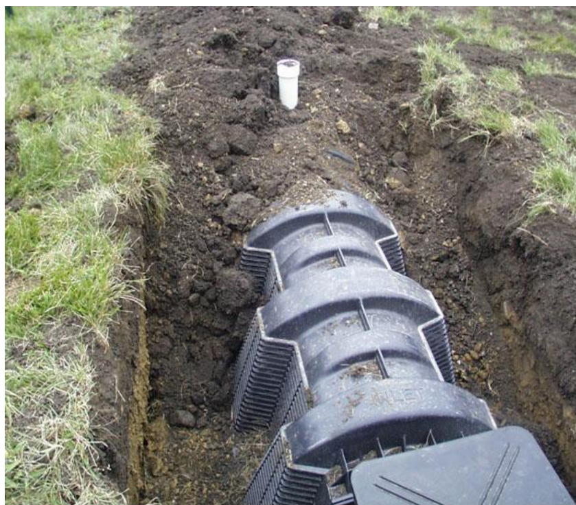
Chamber trench system
